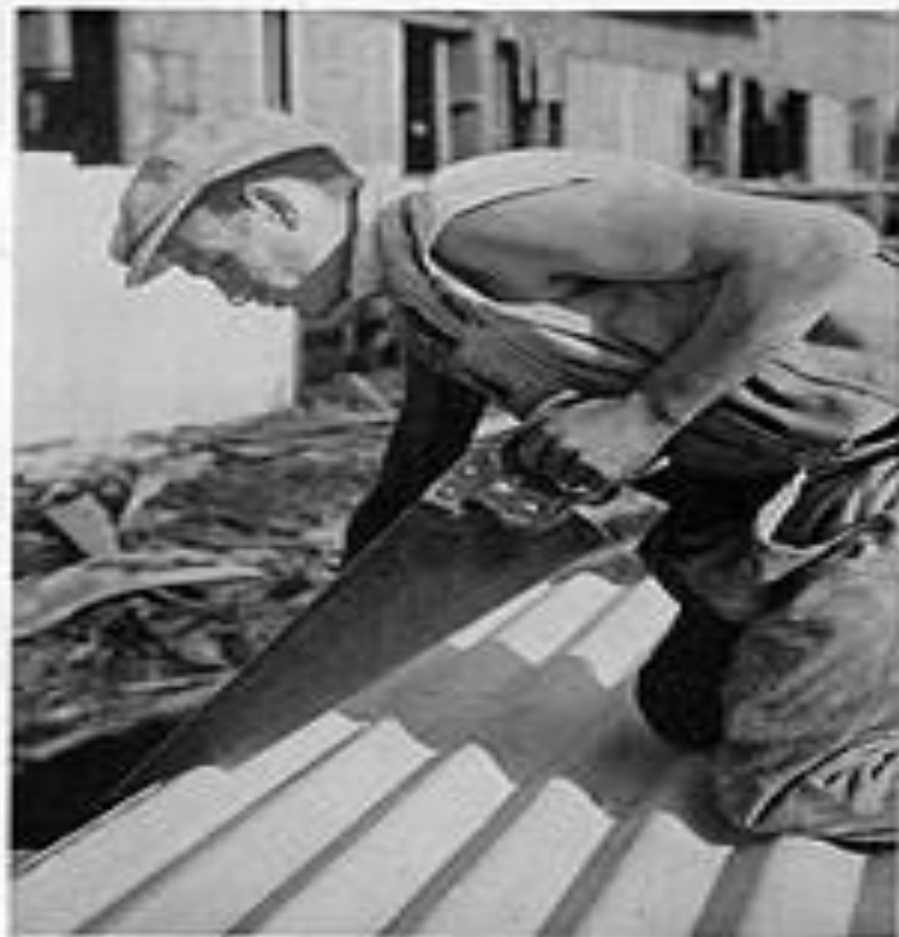
Transite can also be cut with a hand saw
